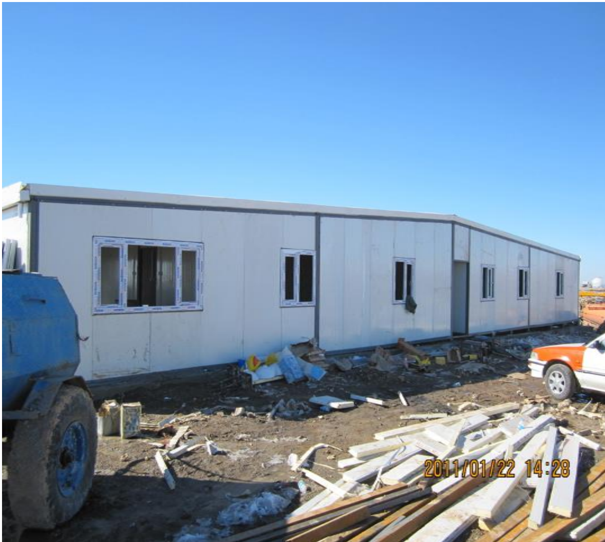
Construction Of Bedroom Hall For OMV Co.
