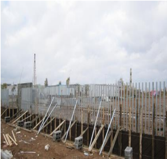
Construction of VAN ROYAL Hotel fence
