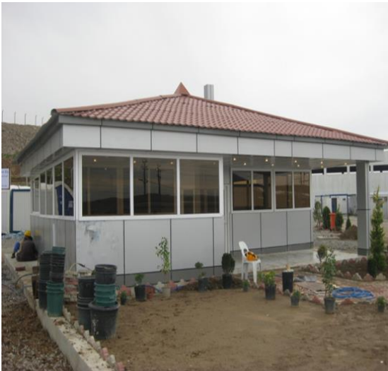
Construction of Mosque In Erbil Refinery
